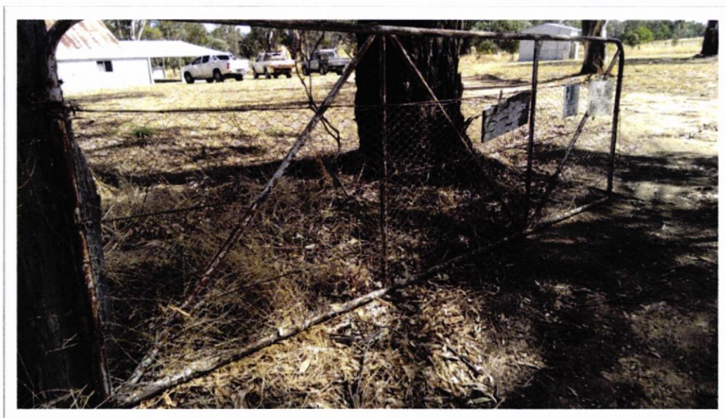
Image 1: Original steel framed gate and signs within the rural fence. The gate is an important aspect of the site and worthy of retention.
