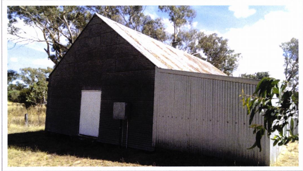
Image 90: The end elevation near the boundary showing the gable ended and the supper room extension. Note horizontal wall cladding and original end door.
