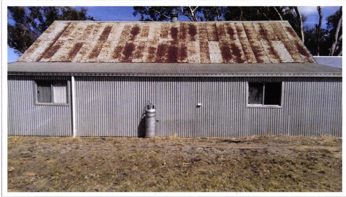
Image 112: The side elevation to the entrance area, noting the supper room extension and original roof behind with central vent cowl.
