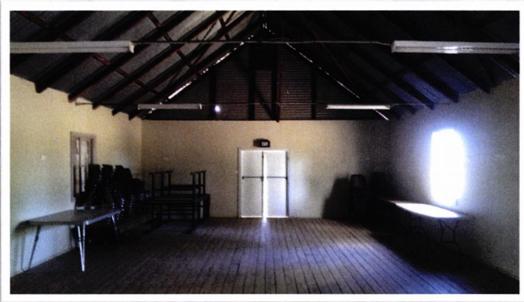
Image 21: General view of the hall interior, noting the roof structure
