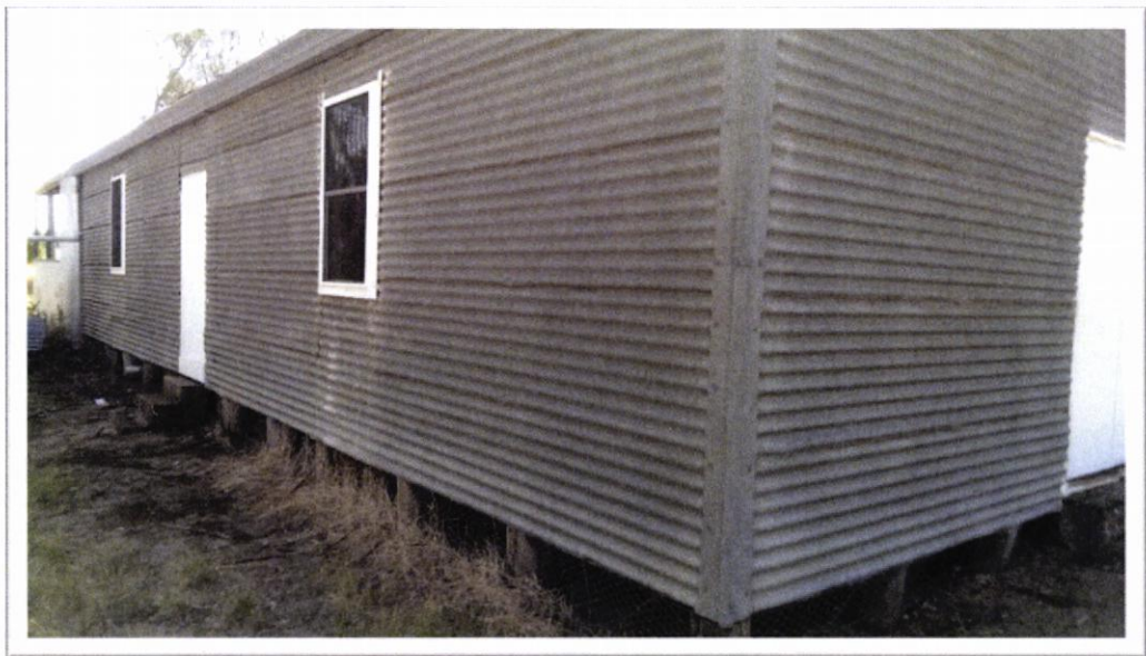
Image 19: The side elevation showing the two replacement windows and original escape door.
