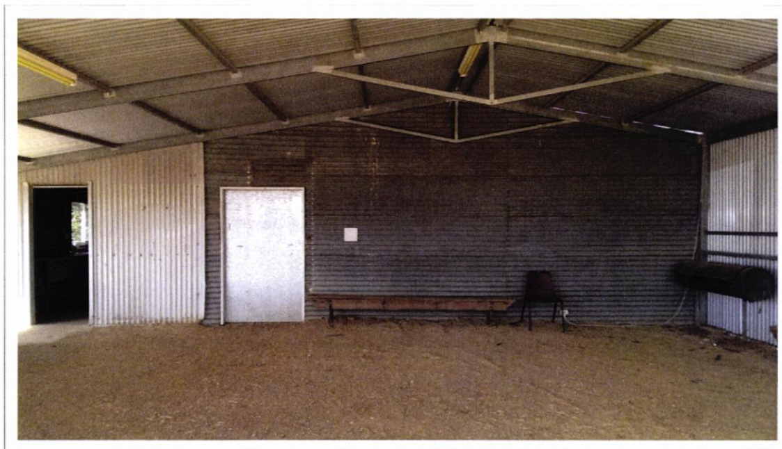
Image 134: View of the main elevation now concealed by the outdoor shelter
